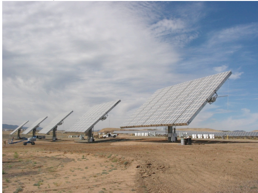
175 kW Amonix Installation at APS
