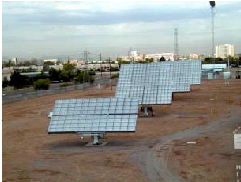
Part of an array field — note the two MegaModule system (10 kilowatt) in the foreground — the MegaModule configuration allows maximum flexibility in field layout
