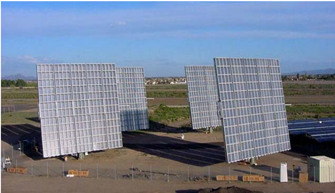
Figure 1. 100 kW of 25 kW arrays installed in Glendale, Arizona in 2001.
