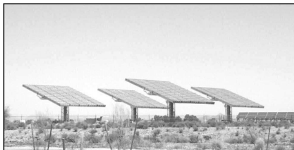
Fig. 2. 100 kW Amonix HCPV at Glendale Airport, AZ
